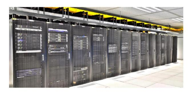
A data centre is a facility designed to house computer systems & associated components such as telecommunications & storage systems. It generally includes redundant or backup power supplies, redundant data communication connections, environmental control (i.e. air conditioning & fire suppression) & security devices. All of these systems ensure 99.99% uptime, 24/7/365 days a year.
